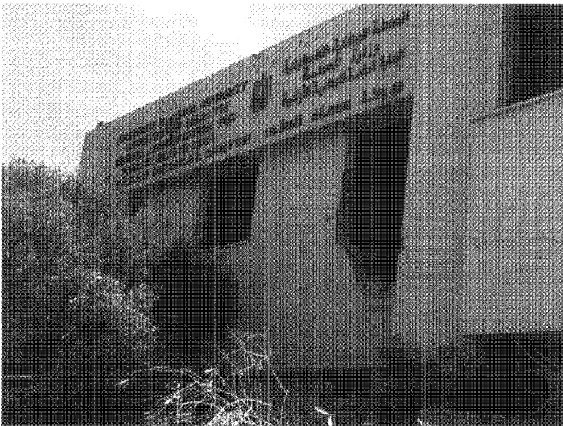
Figure 11: The Palestinian Authority health clinic under which an explosive device was hidden. Damage from the detonation is visible on the clinic's exterior.
